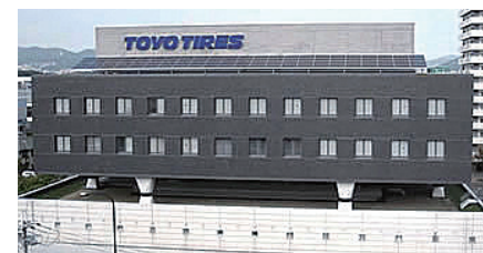
Tire Technical Center with solar panels on the rooftop (Itami City, Hyogo Prefecture)
