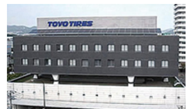
Tire Technical Center with solar panels on the rooftop (Itami City, Hyogo Prefecture)
