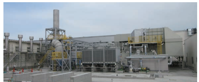
Gas-turbine cogeneration system introduced at the Sendai plant
