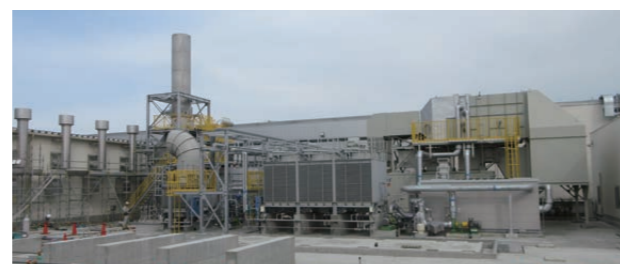
Gas-turbine cogeneration system introduced at the Sendai plant
