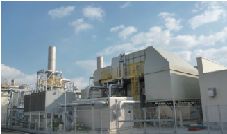
Gas-turbine cogeneration system introduced at the Sendai plant
